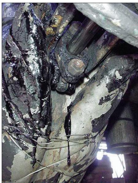
**In comparative testing in a coker plant, 71% of block valves with the 'old' packing were found to leak after seven days as opposed to 16% packed with a new material.**
